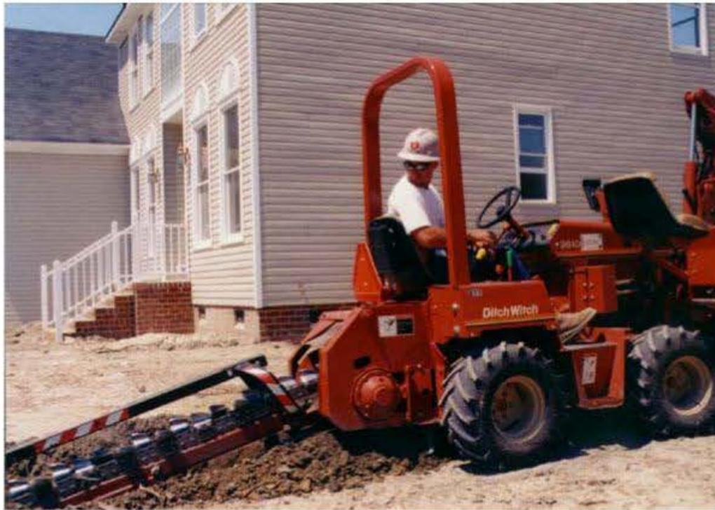
**Figure 12: Installing Flexible Conduit in an Open Trench**
